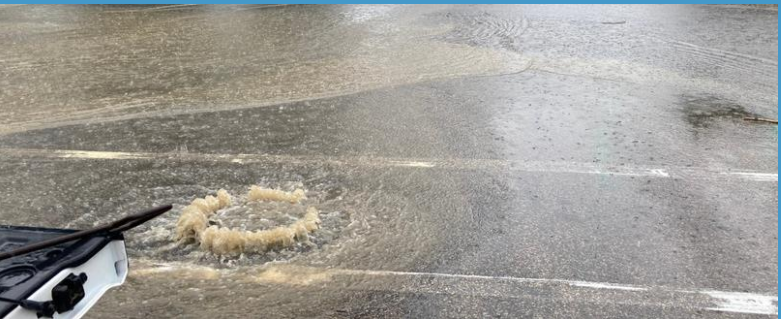
NEAR MALL: BEFORE & AFTER
