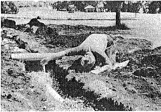
Figure 11. A Local Sanitarian Checking the Depth of Earth Cover Over the Rock. Note the Untreated Building Paper over the Rock and the Distribution Pipe with 1 to 2 Inches of Rock Cover.
