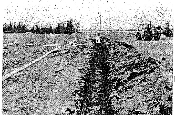
Figure 9. Shallow Absorption Trench After Digging and Before Placing the Rock. The Trench Floor Must be Level Along it's Entire Length.
