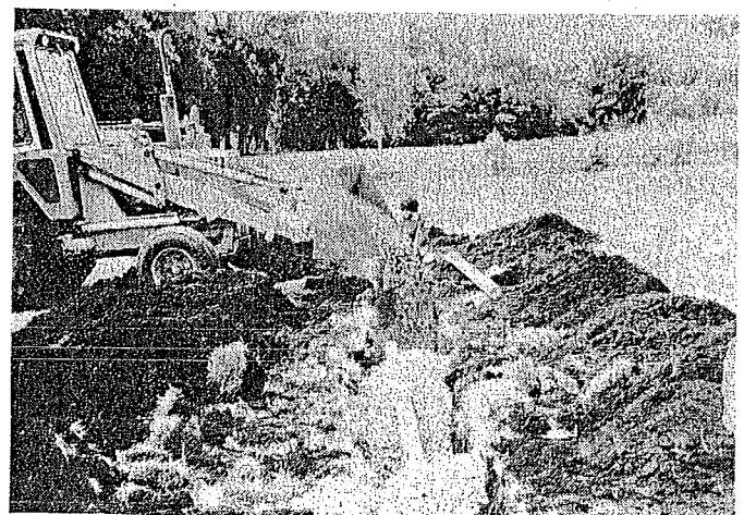
Figure 10. Placing Rock in Trenches With a Front End Loader. The Distribution Pipe is Being Set to Grade.
